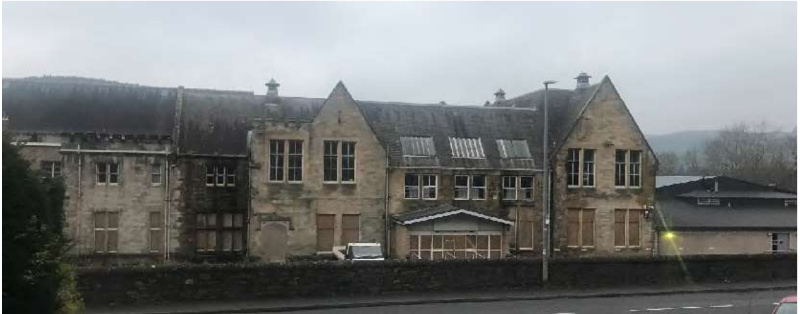
Image 1: Front elevation of former Borders College building
